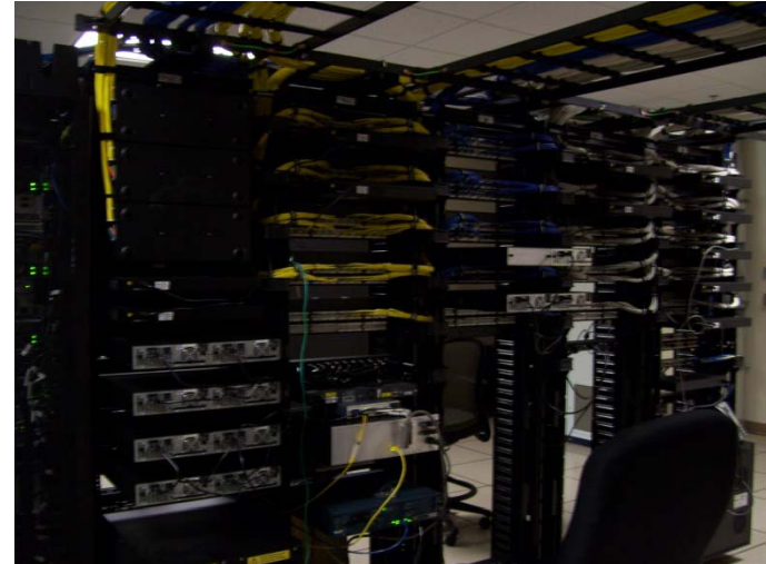
District 4 Palm Beach RTMC Equipment Room
