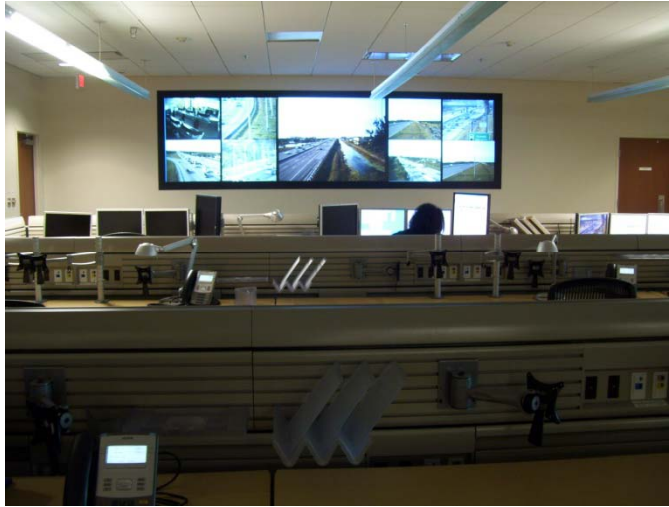
Florida's Turnpike- Pompano RTMC Floor
