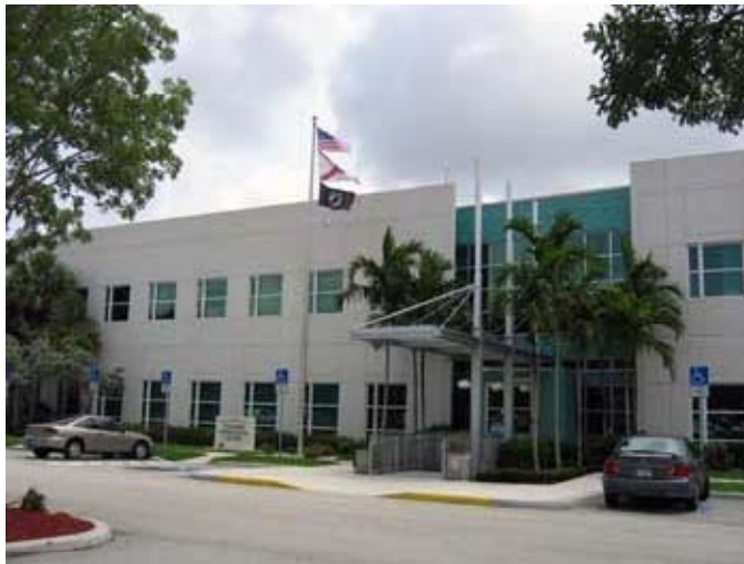
Florida's Turnpike-Pompano RTMC
