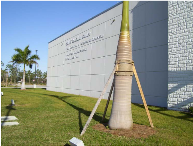
District 1 RTMC Exterior
