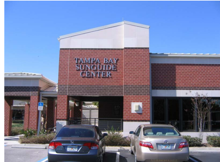
District 7 RTMC Exterior
