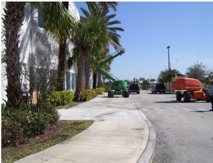
District 6 RTMC Building Repairs
